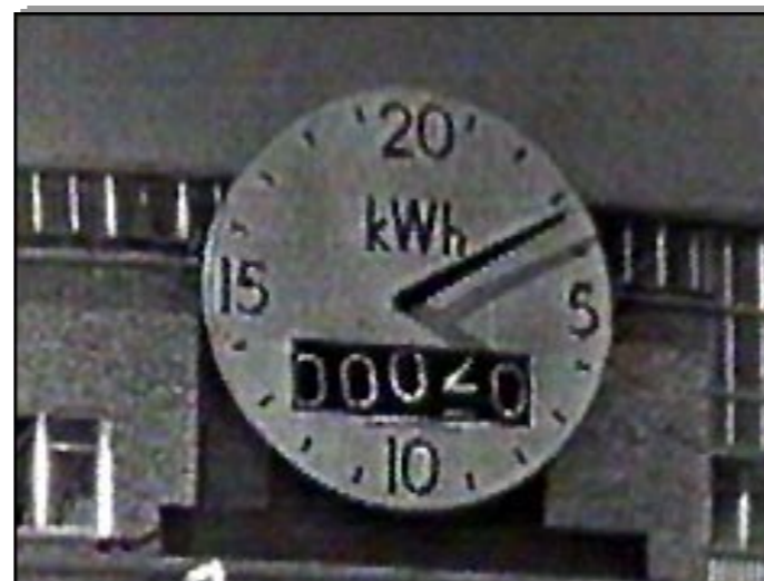
A huge clock registered the first power to be transferred to the National Grid
